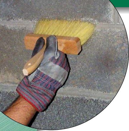
← Applying waterproofing material with a masonry brush.
