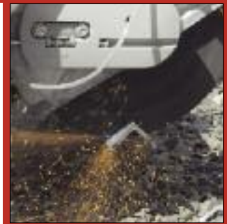
Cutting angle iron with a chopsaw.
